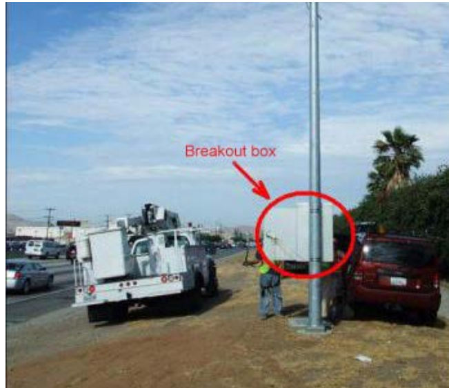
Figure 2-2: Typical Breakout Box Installation
